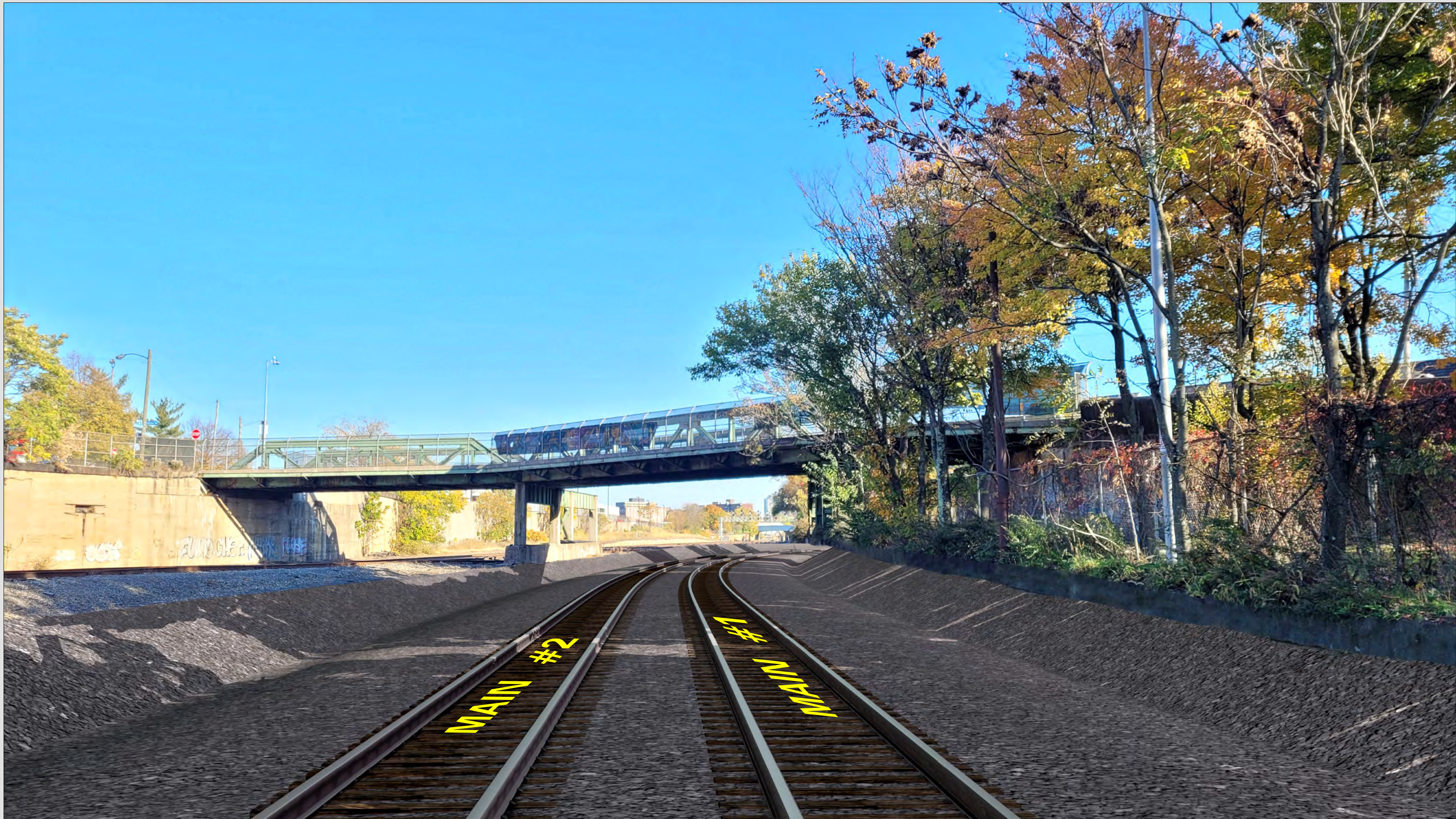
PROPOSED TRACK LOWERING UNDER COLUMBUS AVENUE BRIDGE (OPTION B) FACING SOUTHEAST
