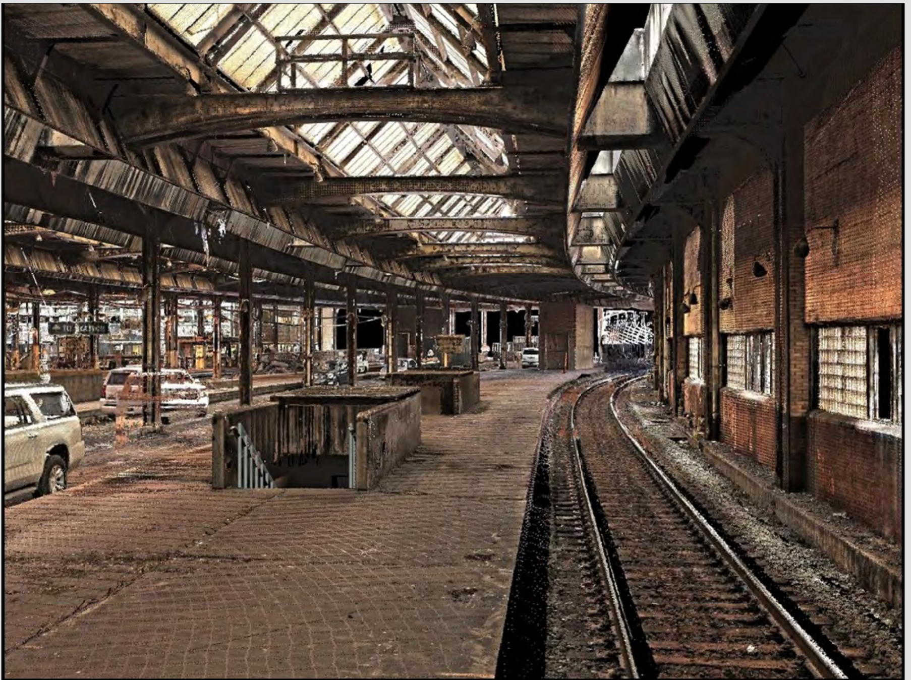
EXISTING GIRDERS AND EXHAUST CHUTES OVER TRACK 2 THROUGH TRAINSHED, FACING WEST
