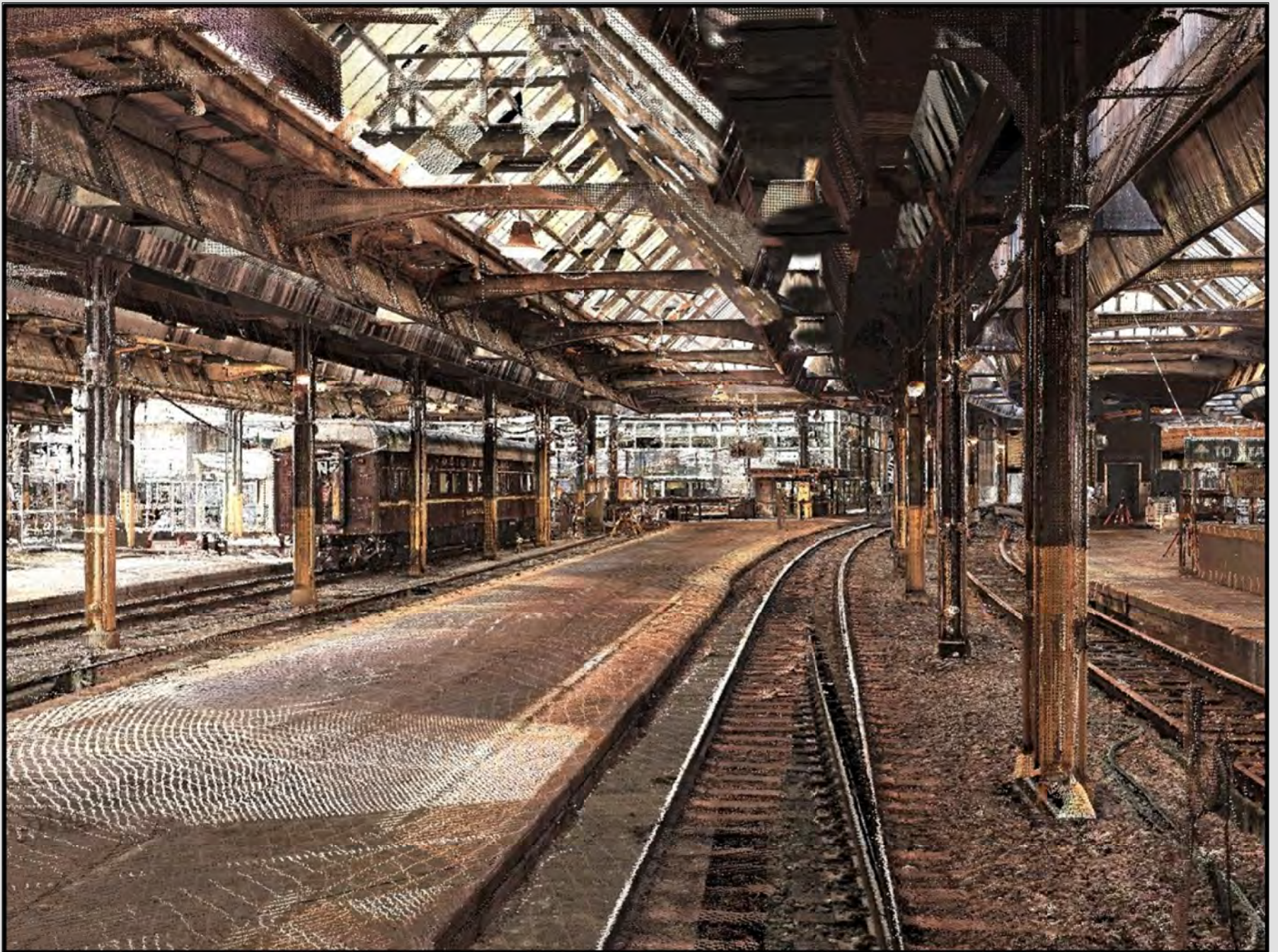
EXISTING GIRDERS AND EXHAUST CHUTES OVER TRACK 1 THROUGH TRAINSHED, FACING SOUTHWEST
