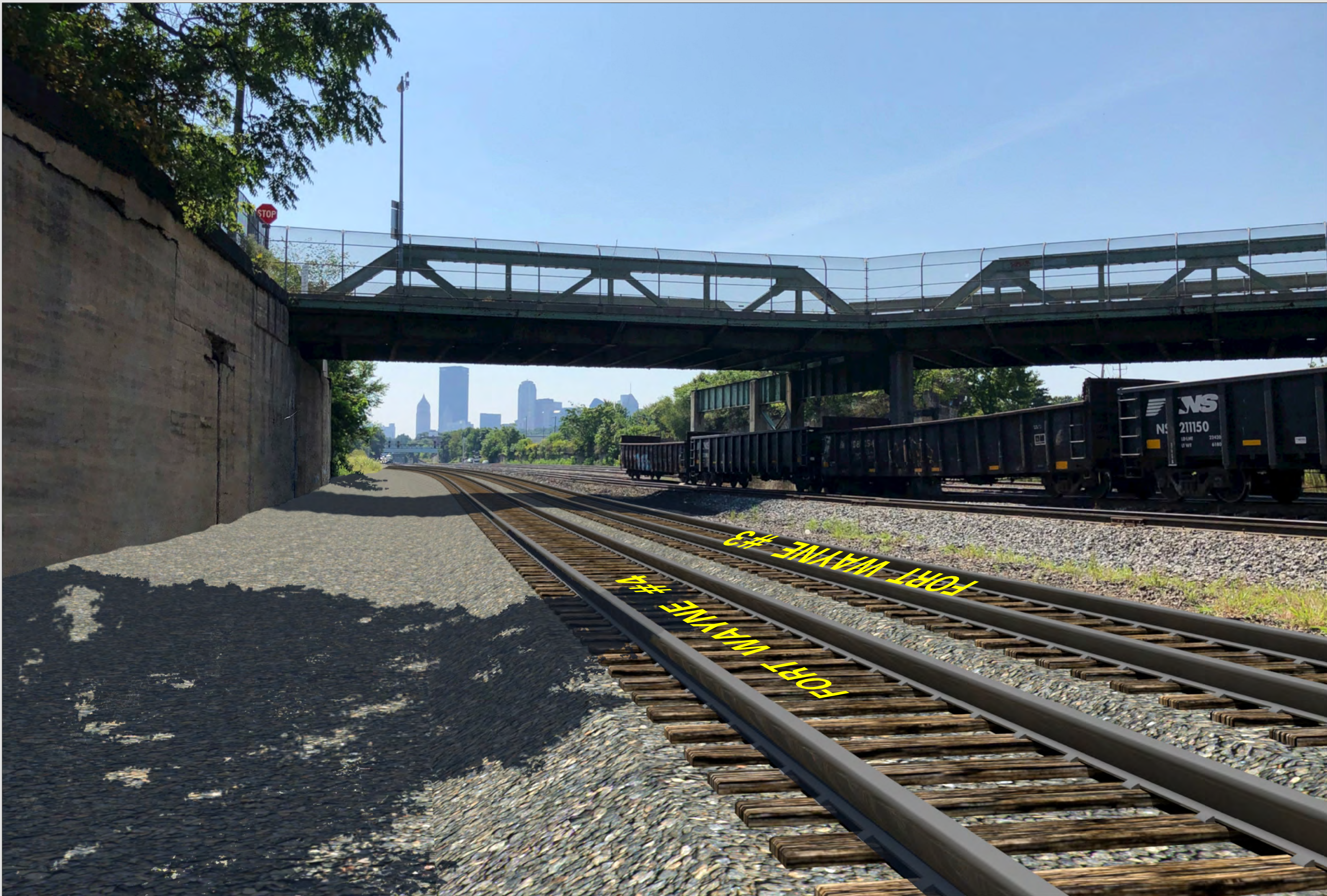
PROPOSED TRACK LOWERING UNDER COLUMBUS AVENUE BRIDGE (OPTION A) FACING SOUTHEAST
