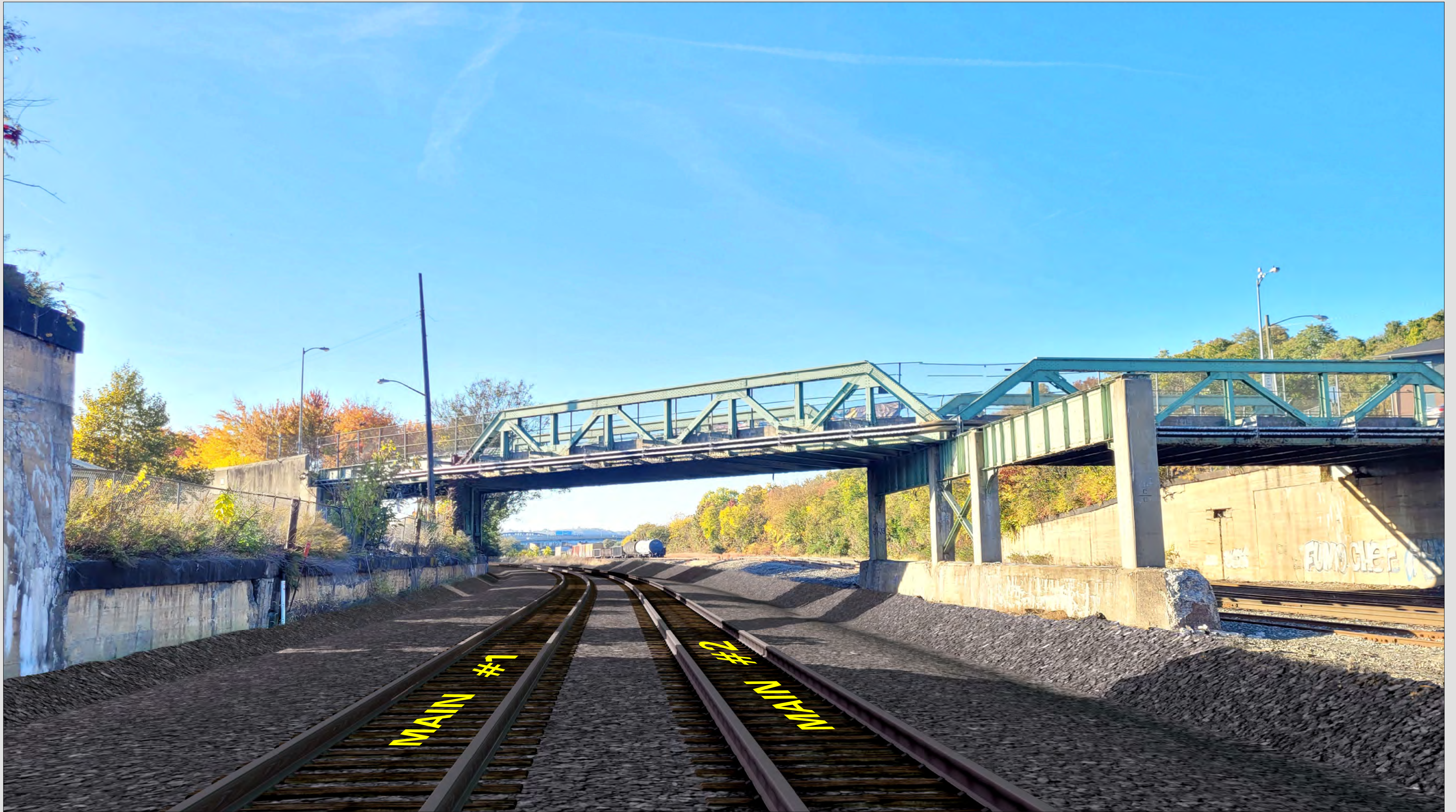
PROPOSED TRACK LOWERING UNDER COLUMBUS AVENUE BRIDGE (OPTION B) FACING NORTHWEST
