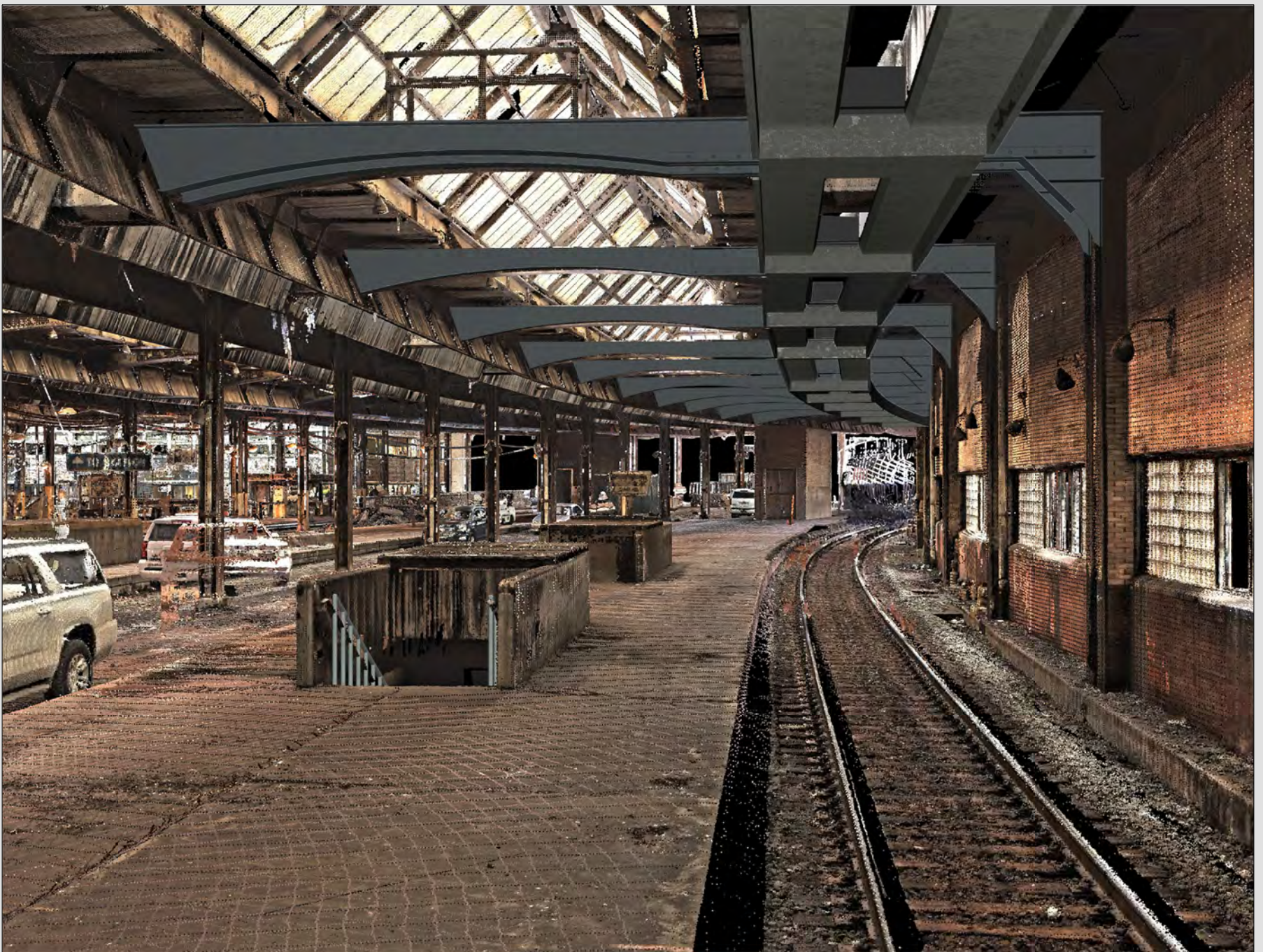
PROPOSED GIRDERS AND EXHAUST CHUTES OVER TRACK 2 THROUGH TRAINSHED, FACING WEST
