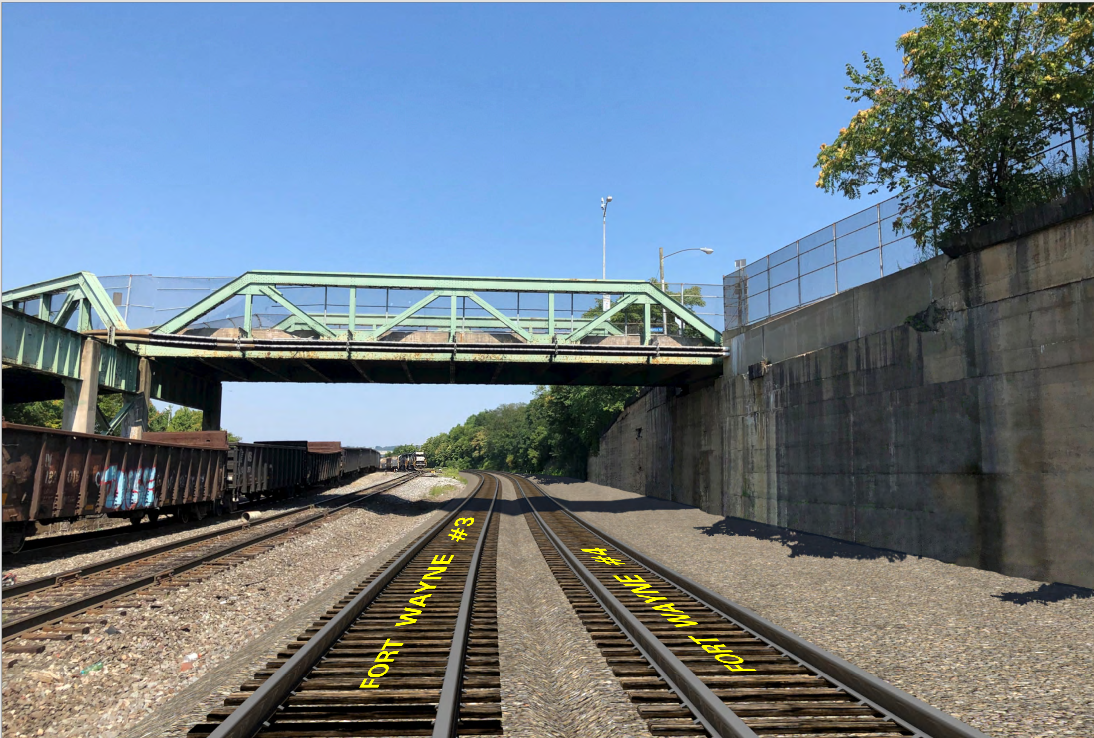
PROPOSED TRACK LOWERING UNDER COLUMBUS AVENUE BRIDGE (OPTION A) FACING NORTHWEST
