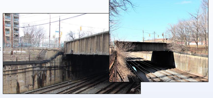
Two small areas of concrete retaining wall with stone coping will be affected by the extension of the northeast abutment. Stone coping will be reused where needed.
