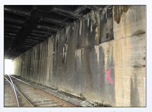
The existing abutments will remain in place; the project will require the abutments to be modified in height and width to accommodate the new bridge superstructure.
