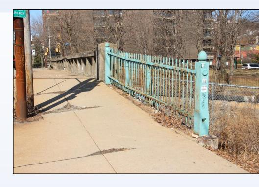
The existing retaining wall and railing along the east side of Brighton Road were constructed along with the 1929 bridge and will be replaced. Because this section of roadway is within the clear zone of the bridge, a safety barrier will be required. It is proposed that the bridge railing match the decorative wrought iron fencing bordering the railroad corridor.
