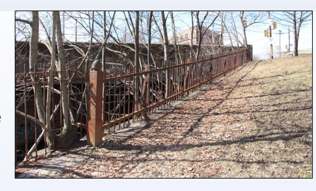
A section of non-matching iron fencing along the northeast side of the rail corridor in the park (replaced in 1929 when the new W. North Avenue Bridge was constructed) will be removed for the extension of the northeast abutment.
